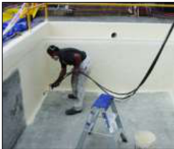
WATER TANK / SUMP
