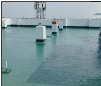
TERRACE WATER PROOFING
