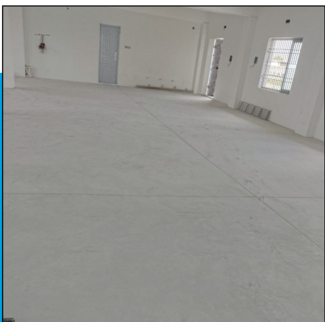
INDUSTRIAL FLOORING WITH POWER TROWEL FINISH
