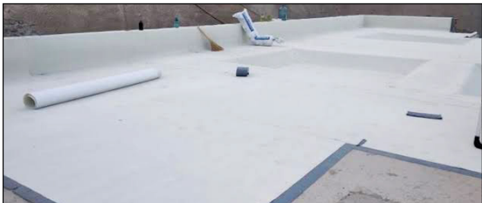
HDPE MEMBRANE BASEMENT FLOOR
