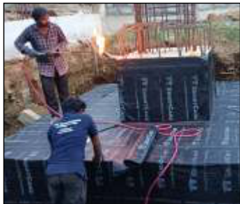
BASEMENT / UNDER GROUND
