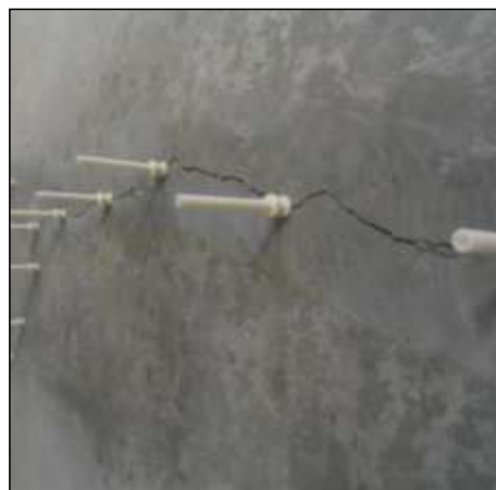
INJECTION GROUTING (CEMENT , PU AND EPOXY GROUT)
